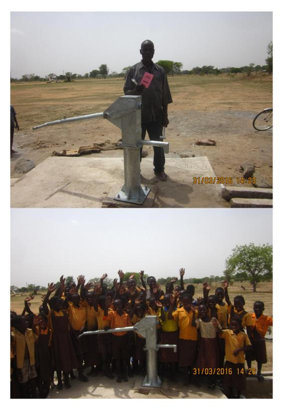
Drilling rig contractor selected, on site, bored for water to 45m, installed and grouted 150mm diameter PVC lining. Set out and constructed concrete pad for pump, with community labour and basic materials, fitted and tested the hand pump.
