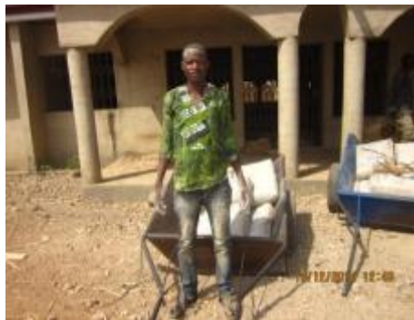
Figure 3 Materials being delivered
