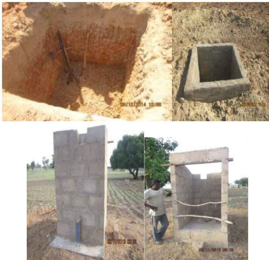
Figure 2 Stages of Latrine Construction
