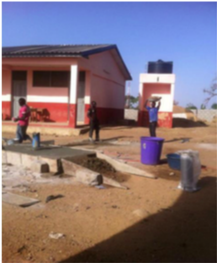
This borehole is drilled by project Bongo and completed by LWA
