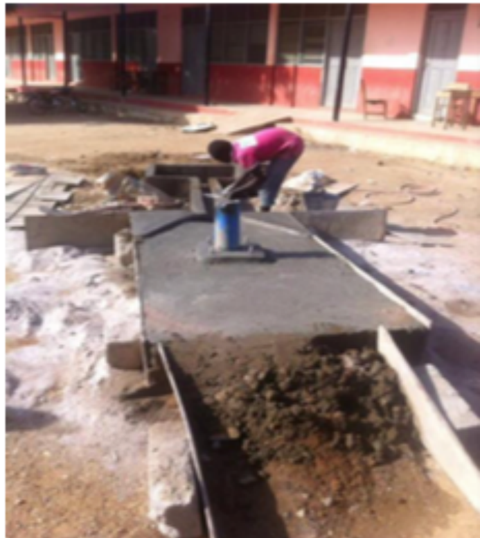
This is Senior High School before – drilled by Project Bongo, Shetland
