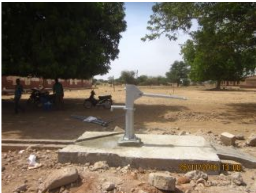
Feo Primary School Before
