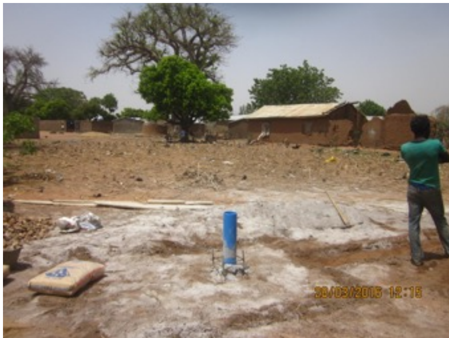
Bongo Central after drilling of the hole, before the hand pump
